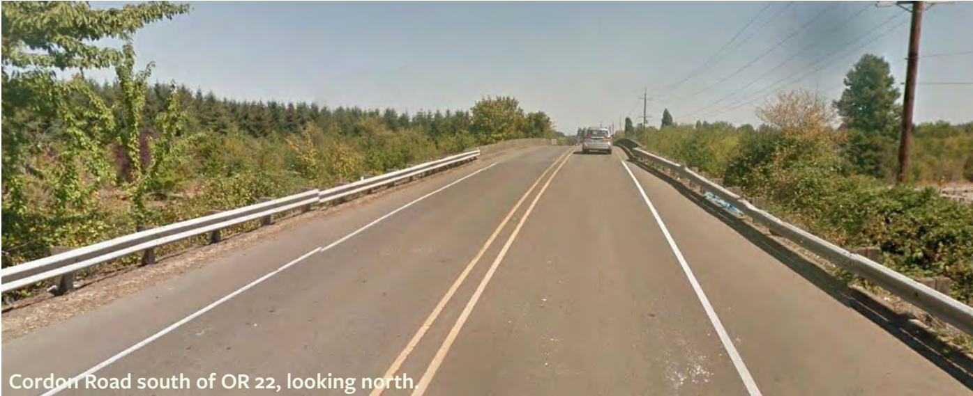
Figure 7. Street-View of Cordon Road Bridge
